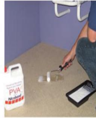
Prime timber and allow to dry
