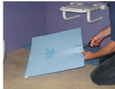
Cut the Plastic Ply using scissors
